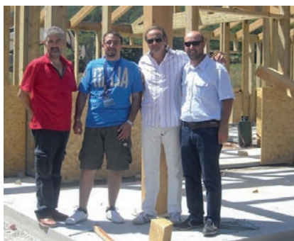
From the left: Fernando Ferrara, secretary of NPO Ambiente e/è Vita; Pierluigi Biondi, Mayor of the Municipality of Villa Sant'Angelo (AQ); Paolo Subissati, CEO of Subissati s.r.l.; Alberto Romagnoli, technical office Subissati s.r.l.
